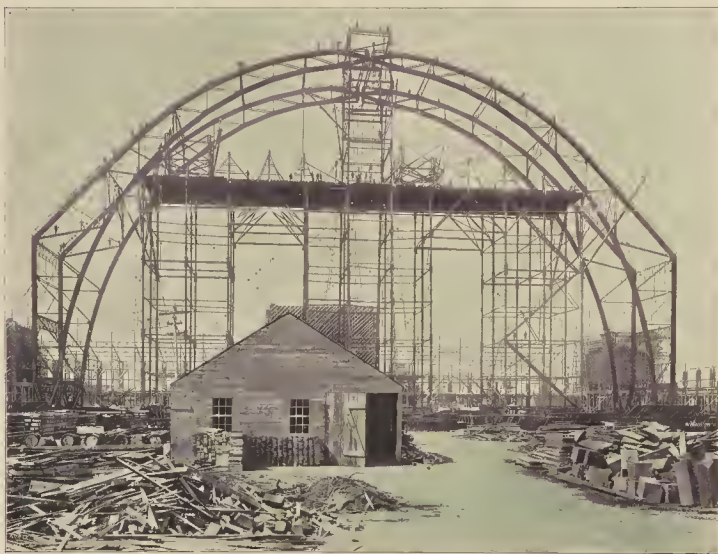
THE FIRST ARCH IN PLACE, MANUFACTURES AND LIBERAL ARTS BUILDING.
